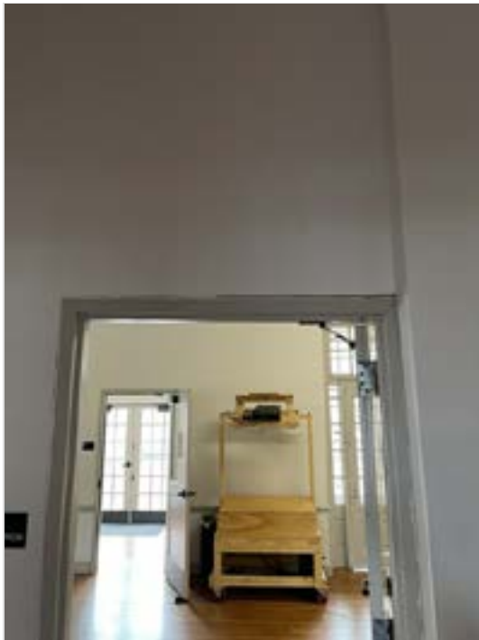
Door frame settling and "detaching" from wall. Remove frame to confirm proper blocking is provided. Reinstall with proper support and paint frame and wall as required.
