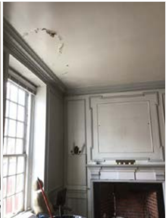
Paint blistering and peeling.
