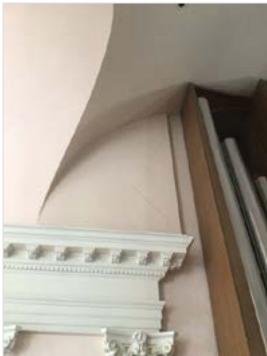
Cracks above decorative wood cornice.
