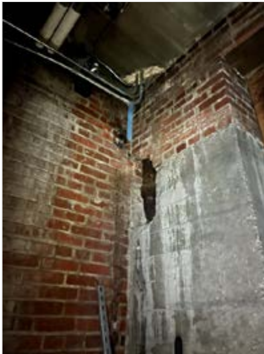
Evidence of water infiltration on masonry walls. Pipe appears to have been previously exposed for maintenance.
