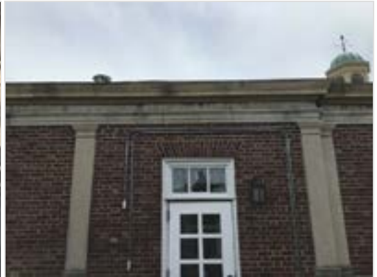
Water damage on cornice
