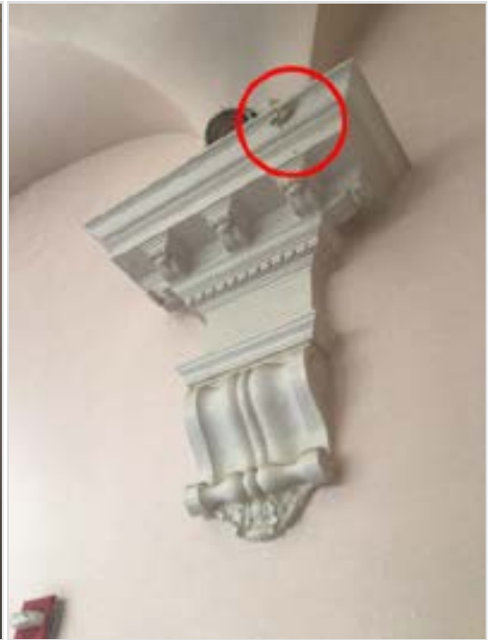
Peeling paint and layer of dust at corbel.
