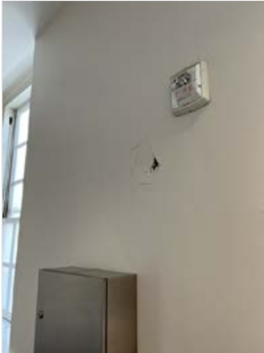
Repair hole in wall for clean smooth finish. Paint as required. Patch paint at restroom sign.
