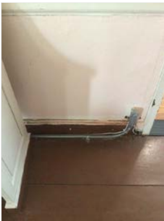
Exposed wiring in multiple locations.
