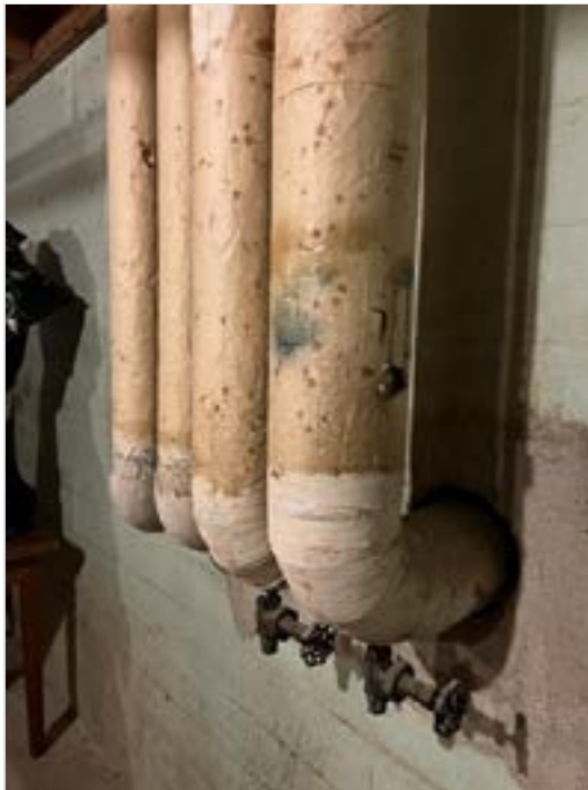
Wear and tear on piping insulation; typical.
