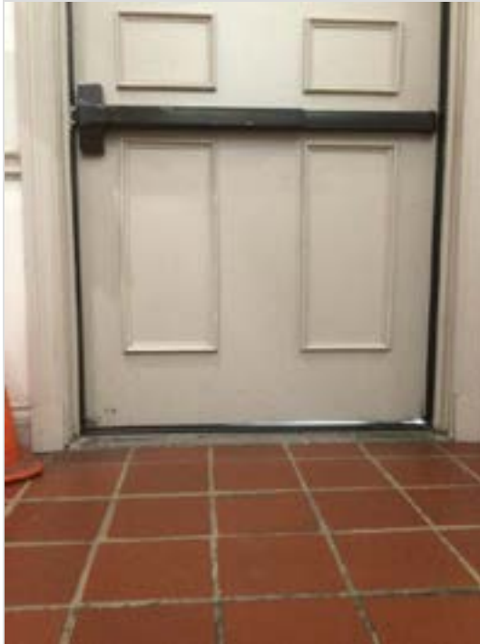
Air gap at bottom of door. Provide proper weather seals.
