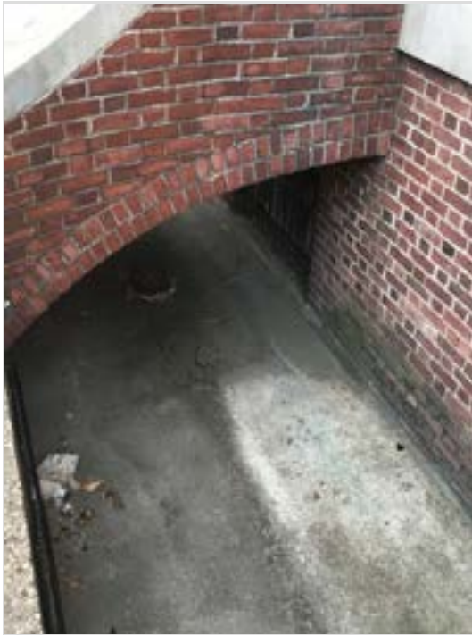
Drain raised above slab + dirt collecting
