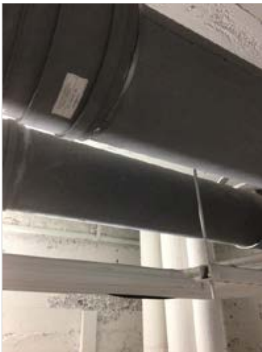
Pipe appears to be leaking at seam. Evidence of leak on floor below. Repair as required.
