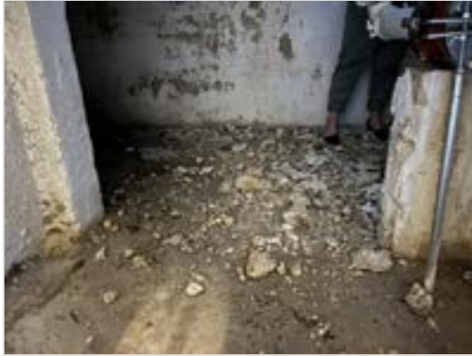
Concrete breaks collected across floor.
