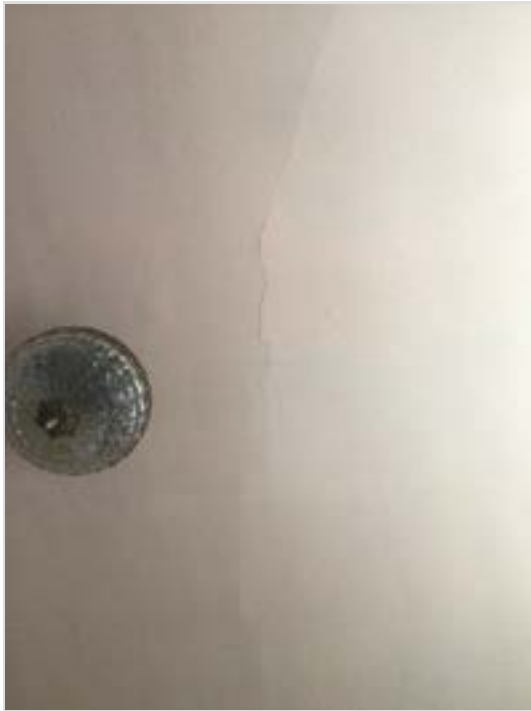
Cracking in ceiling.
