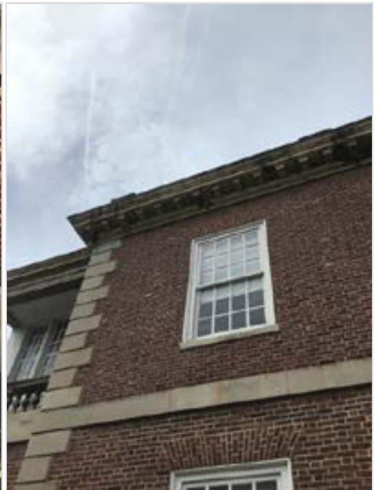
Cornicing has water damage; needs cleaning and gutters may need replacement.
