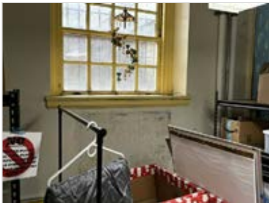
Window sill needs paint, window frame showing signs of deterioration - may need replacement.
