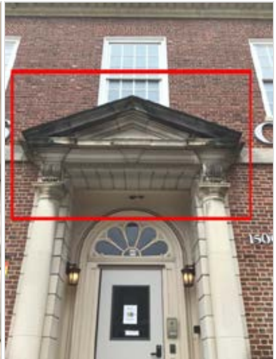
Door in great condition, pediment has significant water damage.
