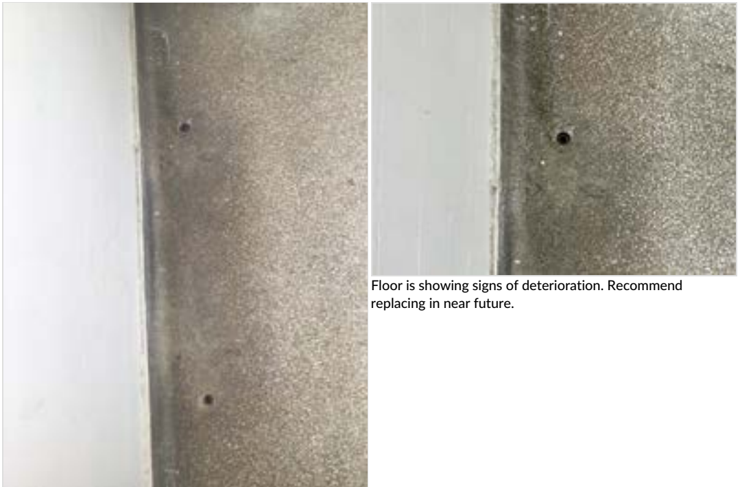
Hole in wood floor.
