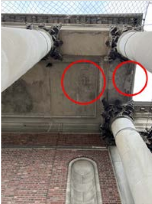
Cast stone ceiling showing signs of water damage / needs cleaning
