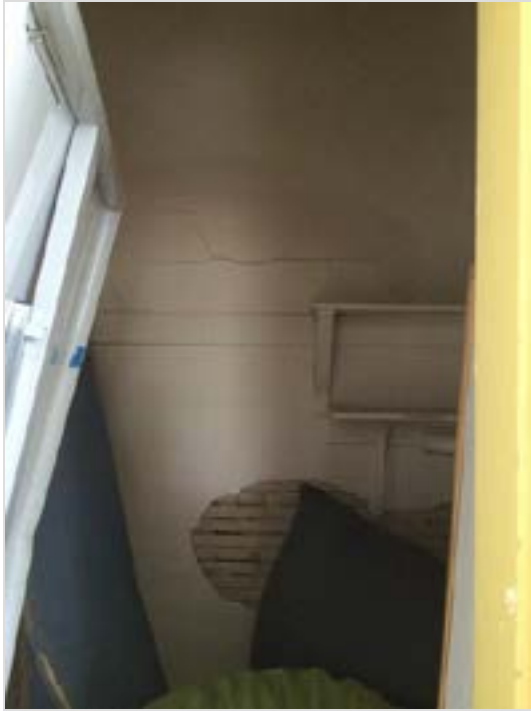
Wall finish in closets are cracking; cause unknown. Further investigation is required.
