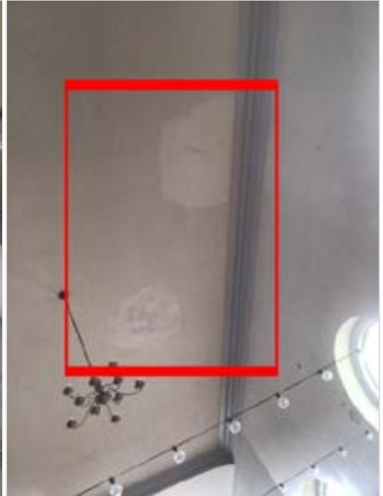
Areas of water damage appear to be painted over.
