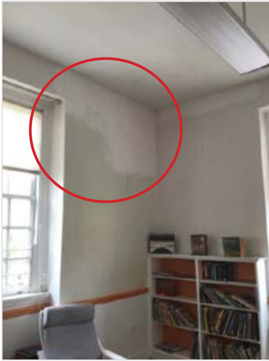
Painting is inconsistent in multiple locations. Repaint room for solid consistent finish.
