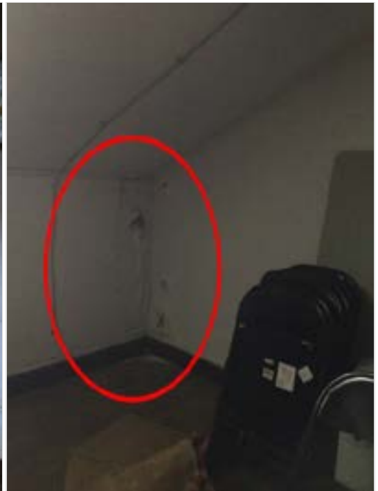
Paint is peeling, chipping & blistering in multiple locations of walls and ceilings. This is typically caused by paint being applied to a dirty surface or fluid pockets. There appears to be no signs of water infiltration. Walls should be repaired/painted.
