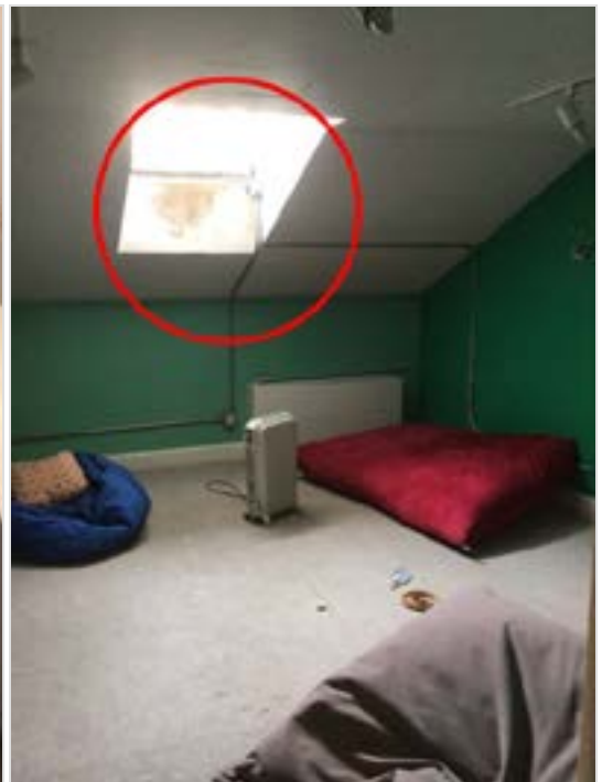
Evidence of water infiltration at window. Investigate source, repair as required and paint wall.
