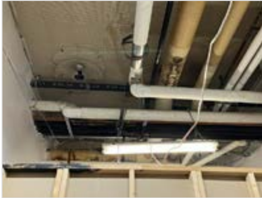
Evidence of water infiltration on pipes and pipe insulation. Investigate for source of leak. Repair leak and replace pipe insulation.
