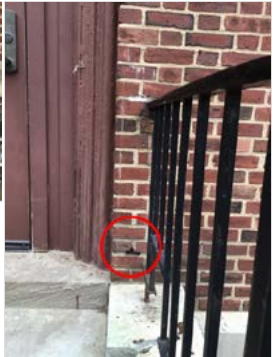
Railing replaced, holes in the masonry left un-filled.
