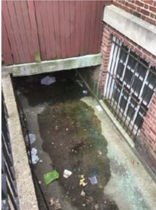
Water collecting under garbage enclosure
