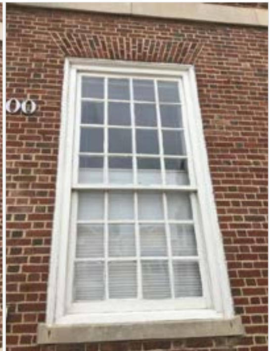
Main level window: paint and weatherstripping may need attention. Window panes and frames will need to be monitored for replacement.
