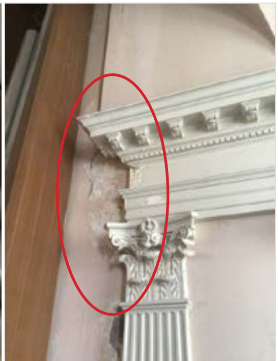
Paint deteriorating by cornice. Cause requires further investigation.
