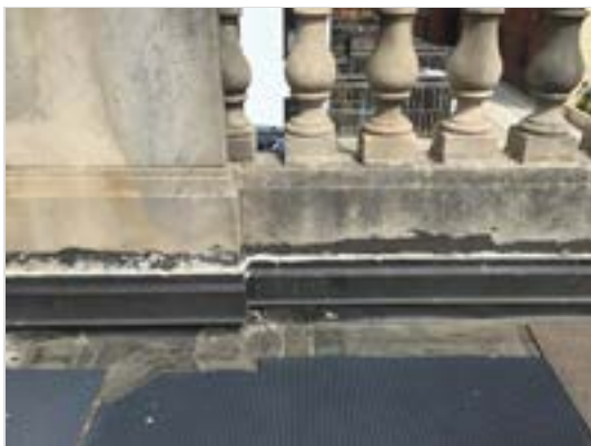
Standing water; slope to drain
