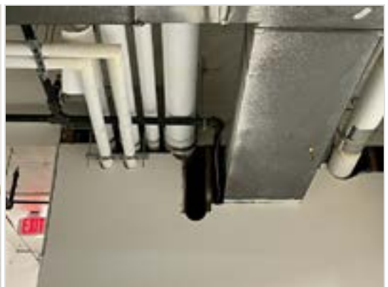
Repair walls around penetrations and paint.
