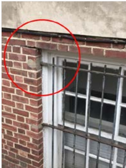
Mortar joint missing near window.
