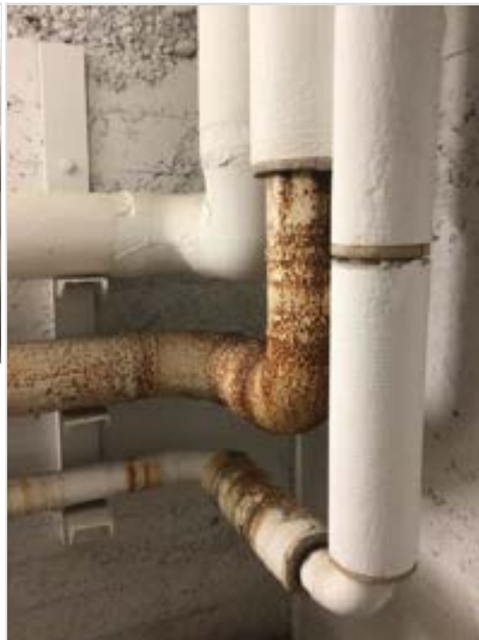
Evidence of pipe corrosion due to water leak. Water leak appears to be from a hot water pipe above.
