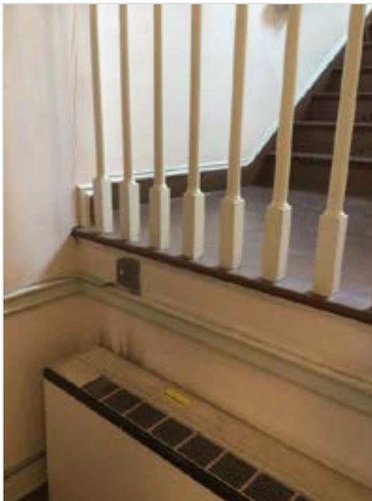
Sand wall smooth. Clean soot from heater. Patch paint and repair wall as required.
