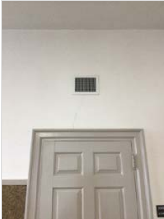
Crack in wall above door. Repair and paint.
