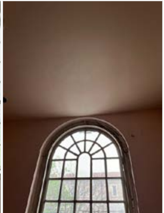
Deteriorating wood frame. Repair and paint.
