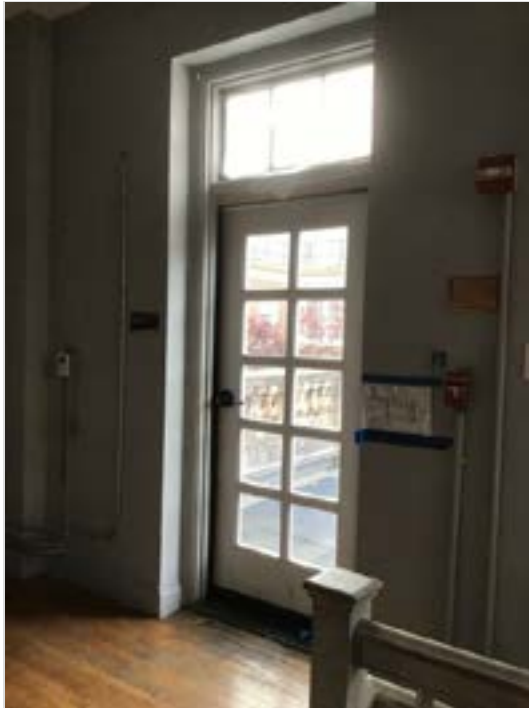
Door does not have weather seals. Seals should be provided. Paint scuffed - paint/clean as required.
