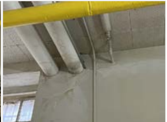
Evidence of water infiltration on pipe insulation and wall.
