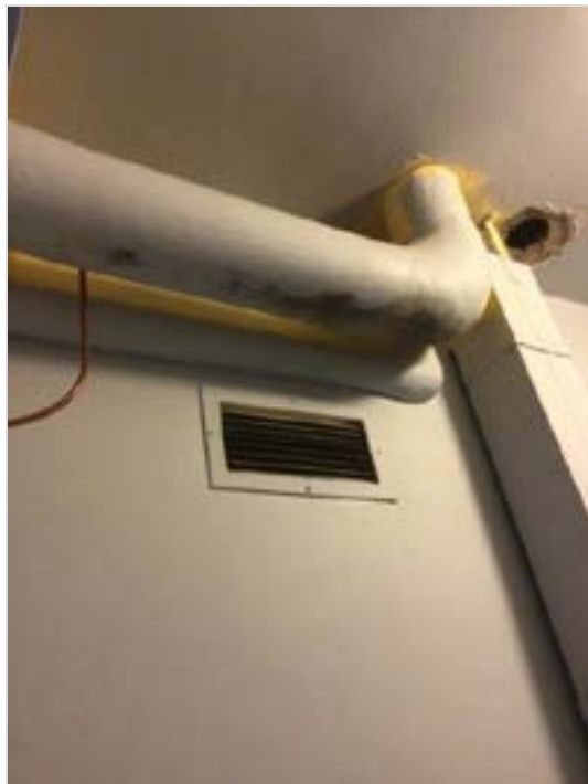
Signs of potential pipe leak due to staining.
