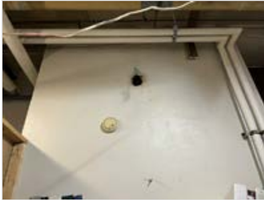
Hole in drywall requires patching.
