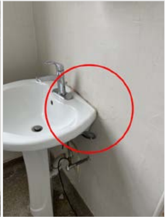
Lavatory pulling away from wall. Re-secure and repair/paint wall.
