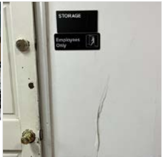
Wood door needs paint; walls chipped and need to be repaired and repainted.
