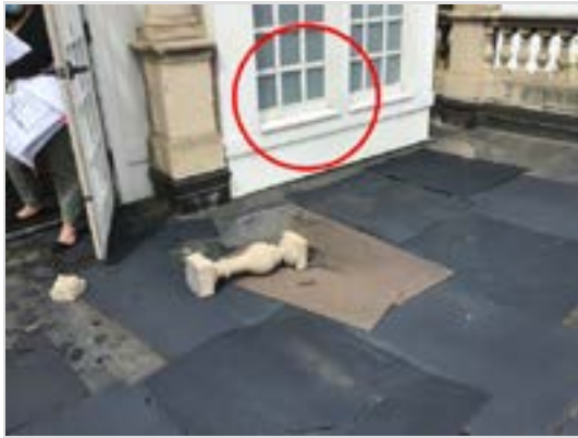
Exposed wood; window frames need repair, refinishing, and/or replacement
