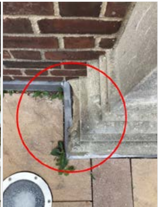
Flashing assemblies need repair at the base of the pilasters.
