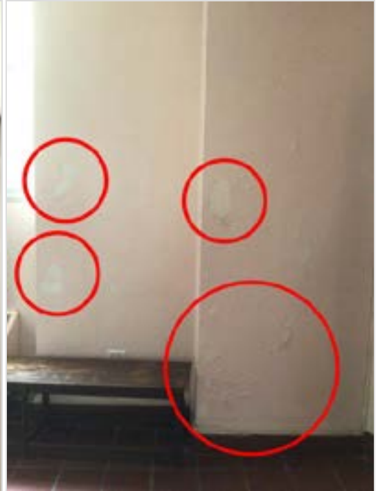
Blistering and peeling of paint.
