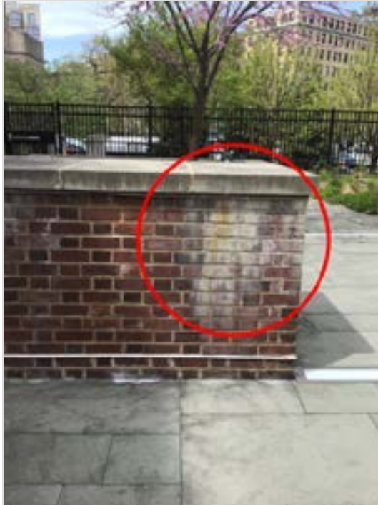
Efflorescence typical on raised brick walls.
