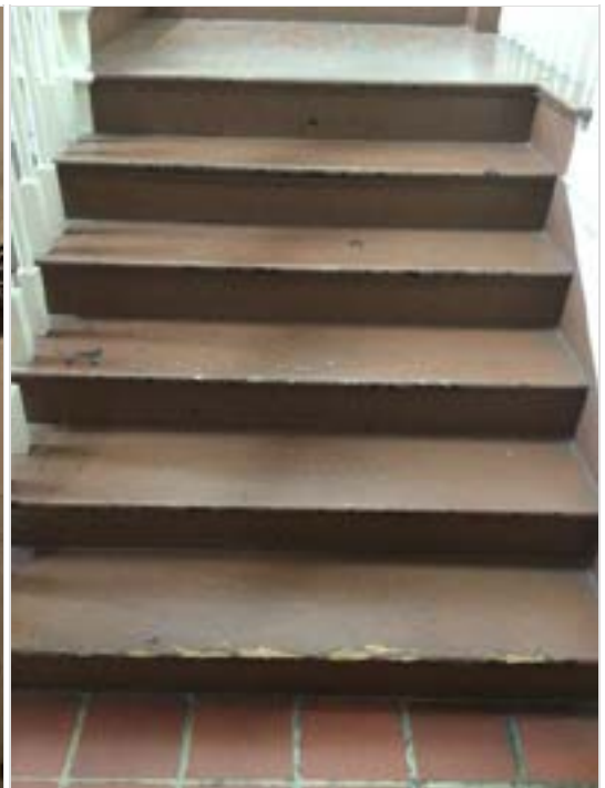
Stair nosings splintering and damaged. Stair requires painting. Rubber surfacing can be applied to tread nosings to help prevent damage of stairs.
