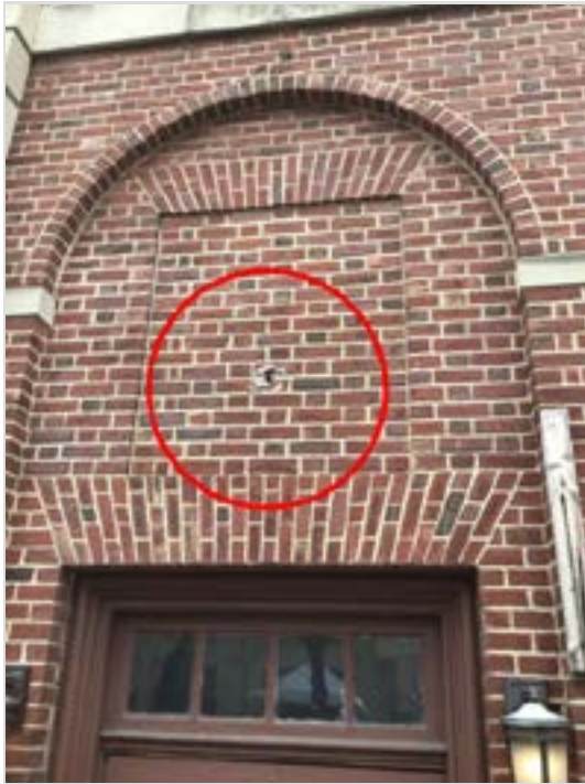
Lighting fixture or flag pole was removed but the hole was not properly filled.
