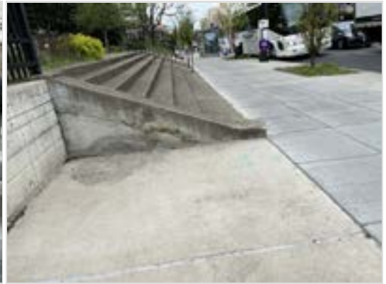
Staircase on 16th street showing signs of corrosion on the concrete.
