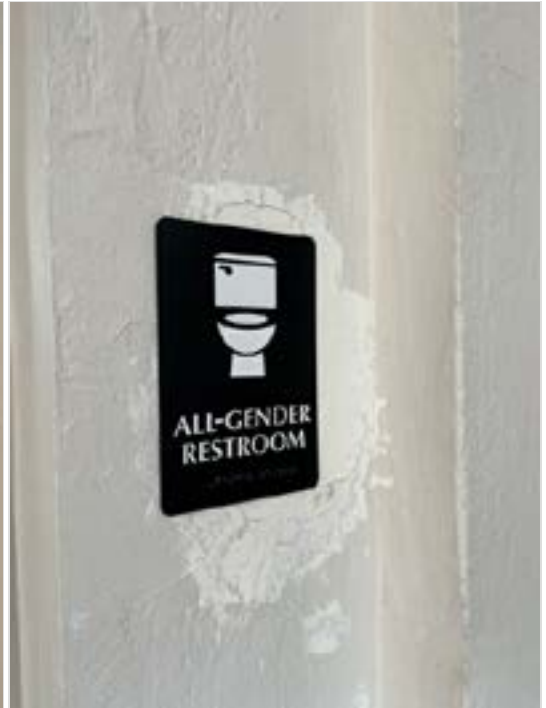
Repair hole in wall for clean smooth finish. Paint as required. Patch paint at restroom sign.
