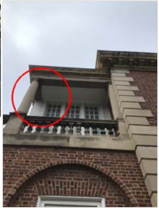
Joint between window wall and masonry portico needs repair.
