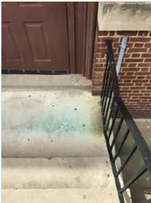
Efflorescence on cast stone directly below the roof line.
