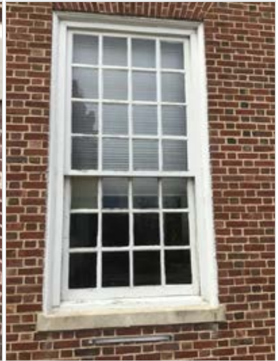
A number of windows on 15th st were not painted in 2015 - - Wood exposed on most typ
