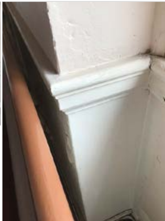
Perimeter wainscoting is chipping. Repair/paint as required.
