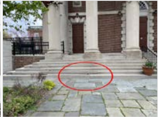
Cast stone stairs not level.
