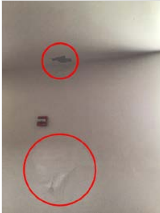
Paint cracking and peeling.
