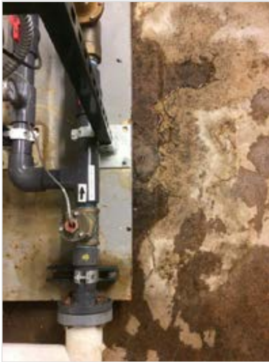
Pump line appears to be leaking from an interior point. Location of leak could not be observed.
