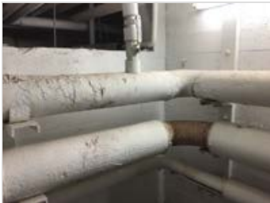
Multiple rips and gaps in pipe insulation. Insulation should be repaired/replaced as required.
