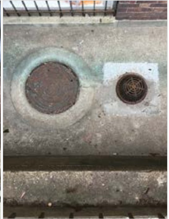
The area below this drain is showing signs of water damage. The efflorescence leads us to believe water has collected here and leaked into the space below.
