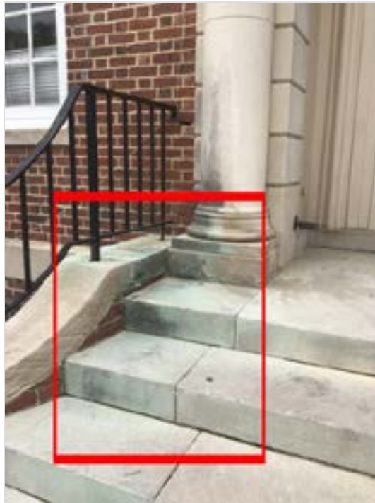
Efflorescence on cast stone steps below pediment.
