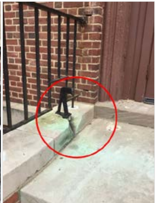
Cast stone cracked
