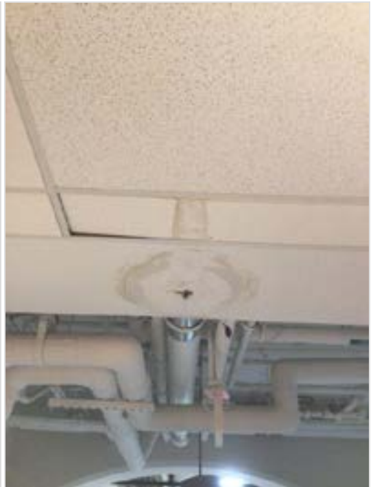
Evidence of water infiltration in ceiling at multiple locations. Investigate above ceilings for cause. Repair/replace ceiling as required.
