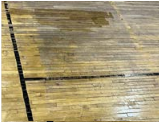
Wood floor is scratched and scuffed. Floor requires refinishing/cleaning.
