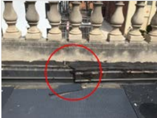
Flashing needs replacement
