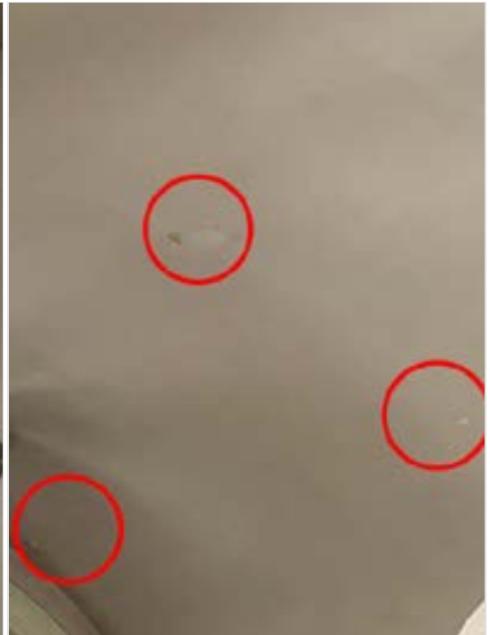
Vaulted ceiling staining and cracking.
