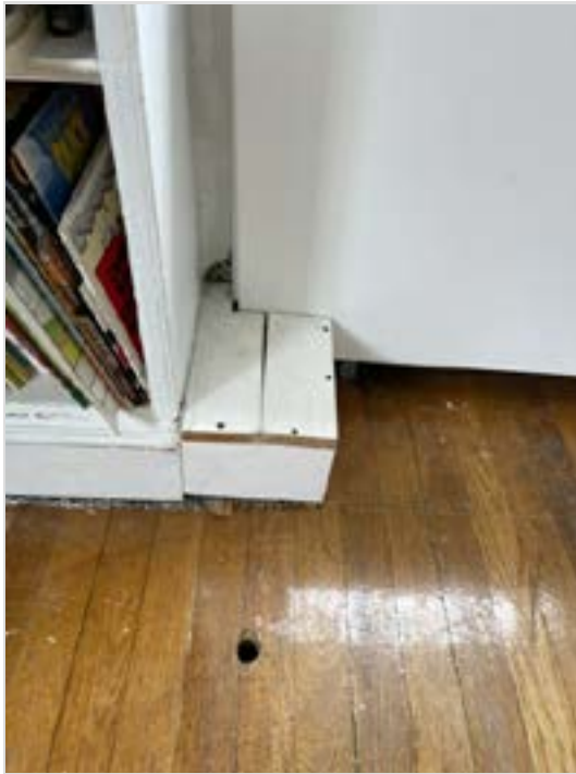
Hole in wood floor.
