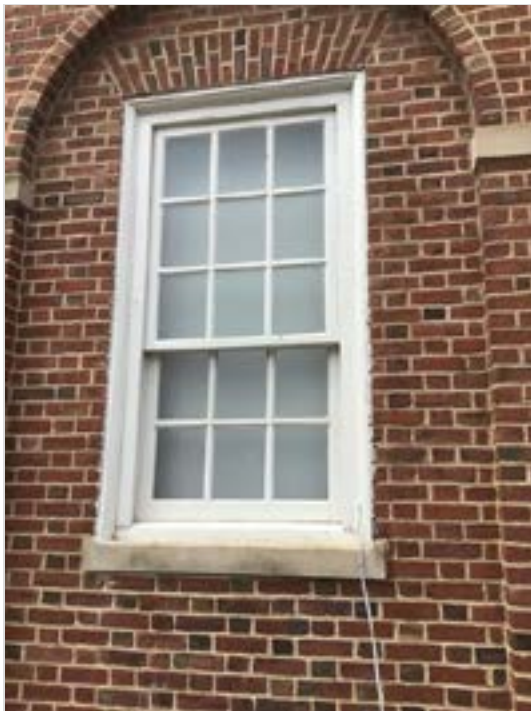
Good window ( restored 2015) Frame needs monitoring
