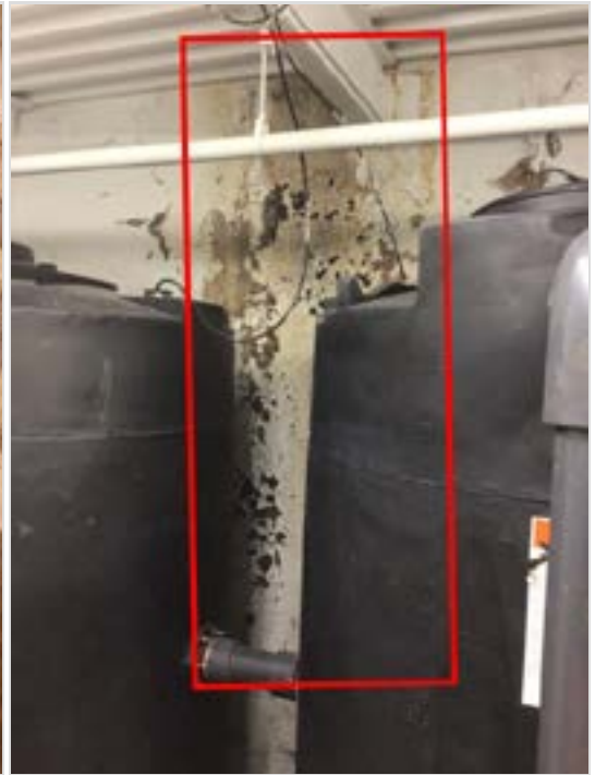
Signs of water infiltration at perimeter wall. Leak appears to be from exterior and will require further investigation to locate.
