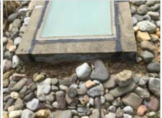
Skylight mortar/ flashing needs immediate attention.
