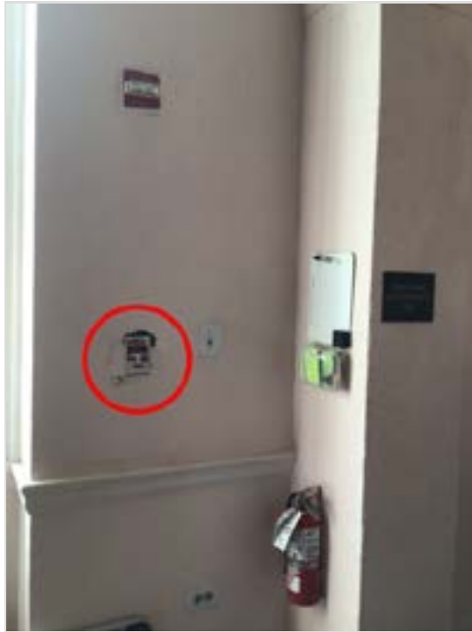
Damaged drywall at fire alarm pull. Repair and paint as required.
