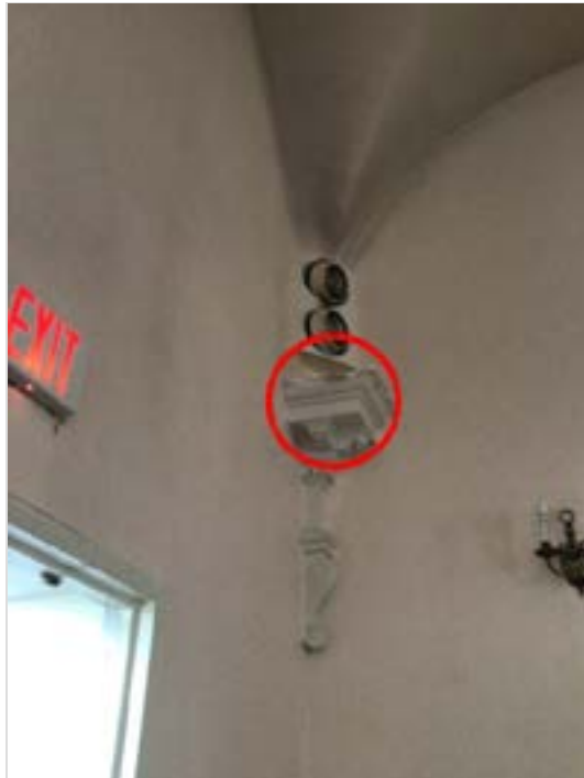
Corbel appears to be deteriorating. Layer of dust visible.
