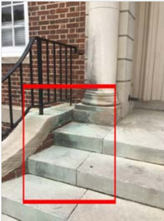
Efflorescence on cast stone steps below pediment.
