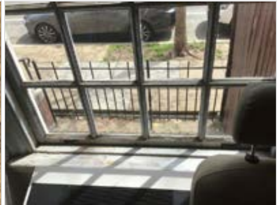
Window requires repainting and weather seals.
