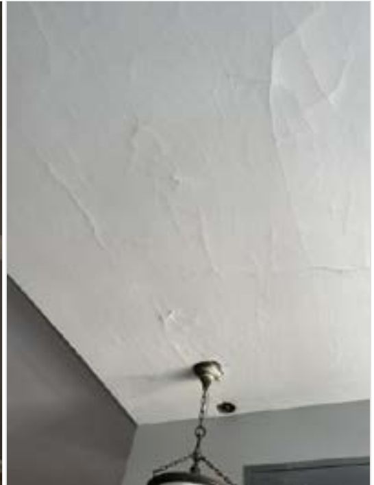
Ceiling paint is cracking. Appears to be due to age and base surfacing. Strip old paint layers and repaint.
