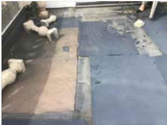
Flexible pavers need replacement
