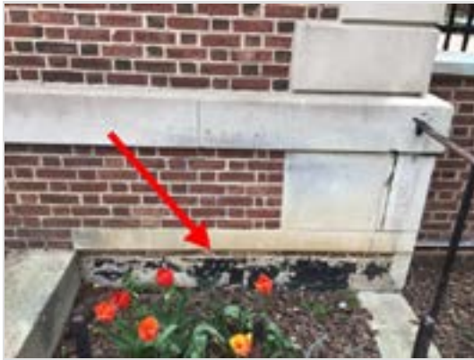
Flashing needs to be repaired at planter on harvard st.
