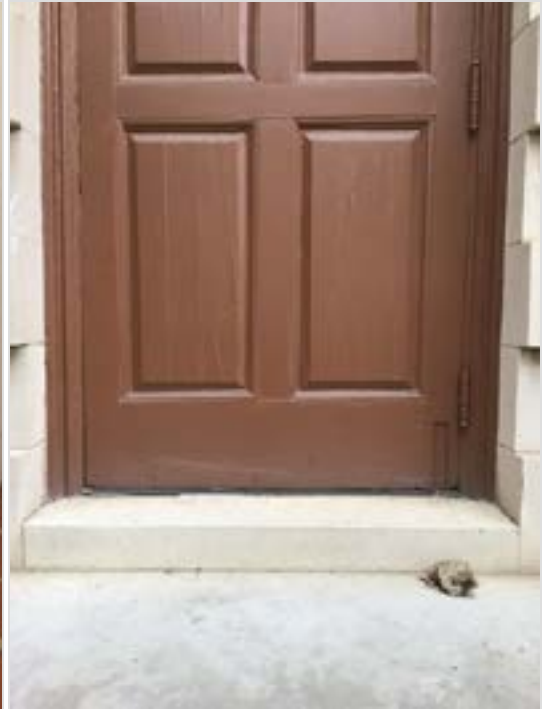
Bottom of wood door damaged. Repair and provide weather seals. A kick plate can help prevent damage to bottom face of door.
