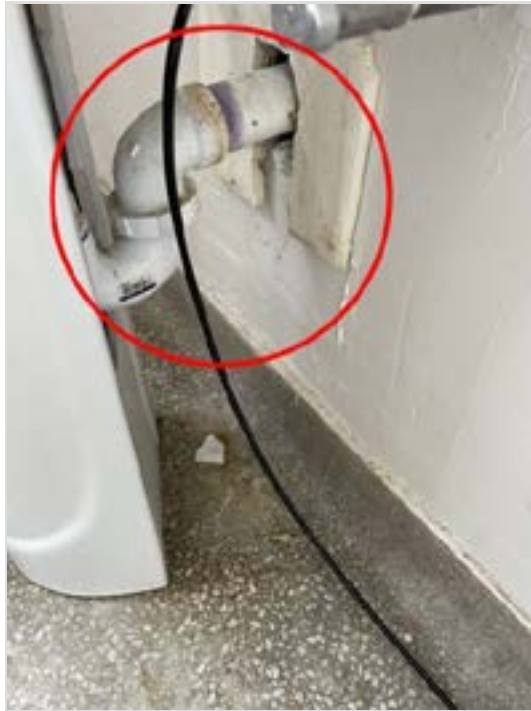
Provide heat shield to keep PVC pipes protected. Seal wall penetration.
