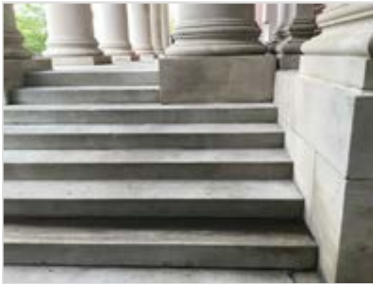
Water collecting on steps to the south west of the front facade.
