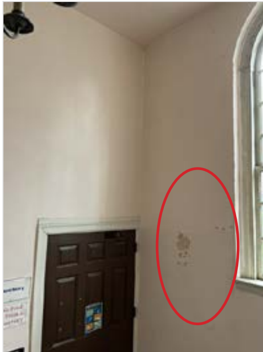
Blistering and peeling paint.
