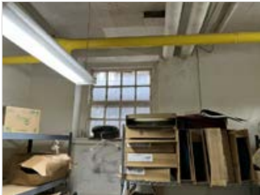
Window frame deteriorating - needs replacement. Window sill needs paint. Walls need patch, repair, and paint.
