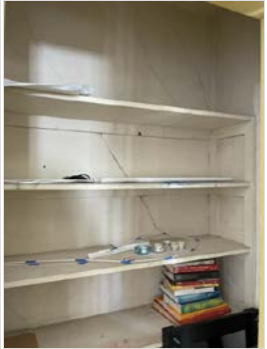
Cracking in closet wall; cause unknown. Further investigation is required.
