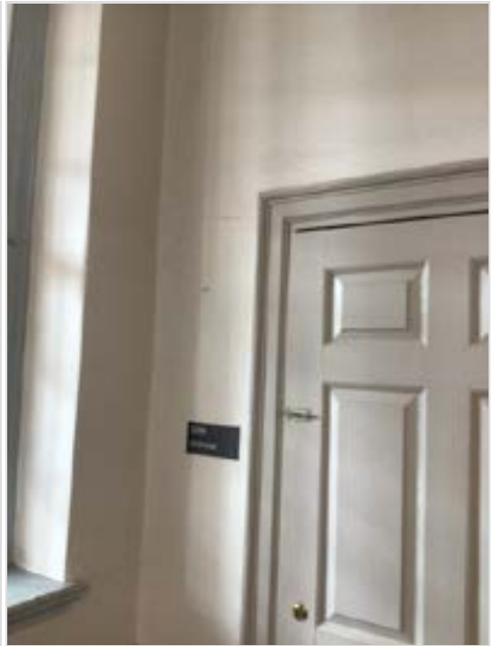
Crack to side of door. Repair and paint.
