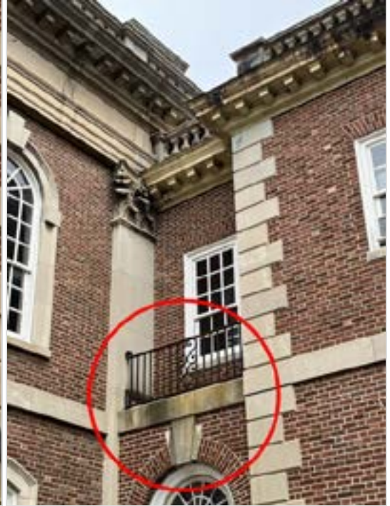
Railing rusting / evidence of water infiltration and damage; investigate and repair.
