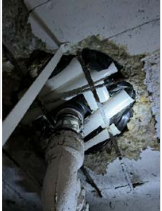
Exposed pipe and main location of concrete deterioration.
