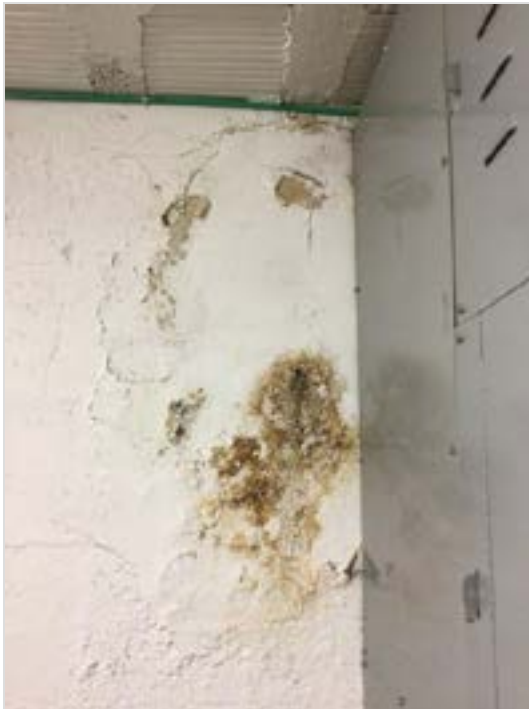
Signs of water infiltration at back corner of the room.
