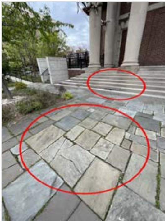
Uneven surface of pavers may not meet accessibility requirement's
