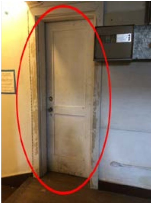
Door to bell tower requires repair and paint.
